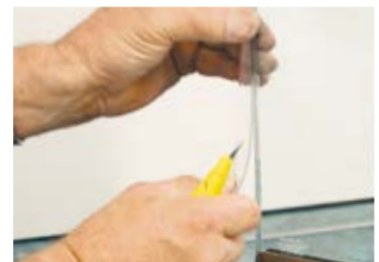
Cut the new and matching water seals to the same length as the originals and install.
