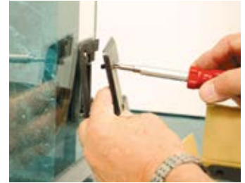
Install a new gasket and interior cover plate, replace screws, then secure in place.
