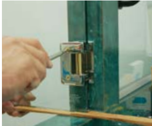
Loosen the cover plate and align the door. NOTE: Make sure Wood Shims are placed under glass to prevent breakage.
