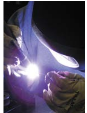
Welding on All Diameters
