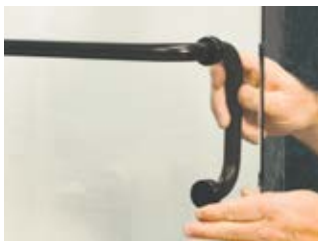
Install the new handle or knob and secure washers and set screws.
