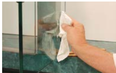
Block the door to maintain alignment and remove the cover plate. Clean glass in gasket area.
