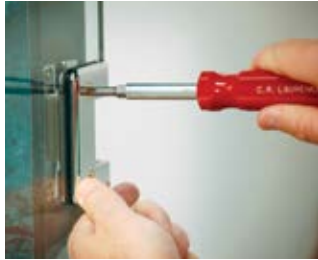
After alignment, tighten the cover plate screws by hand. Do not use a power tool, or you risk damaging the screw heads.
